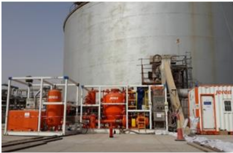
Automatic Hydrocarbon Tank Cleaning
